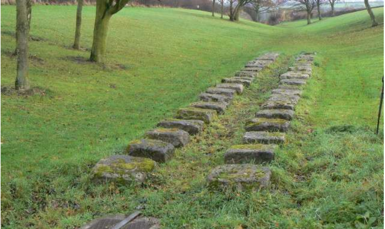
Stone sleepers on Brusselton Incline
