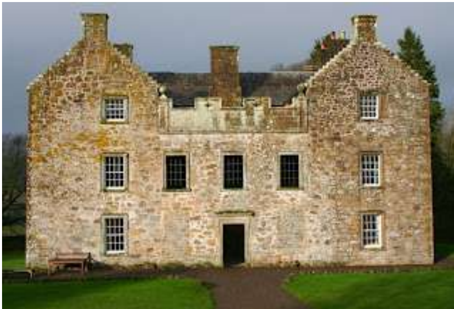
Stonegarthside Hall, Penton (not such a typical house!)
