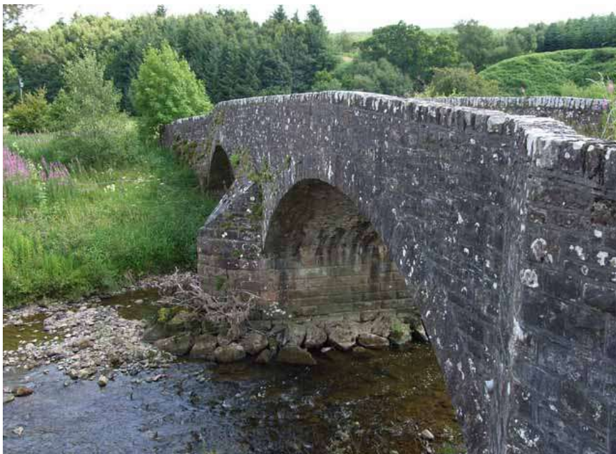
Bridge Over Liddel Water
